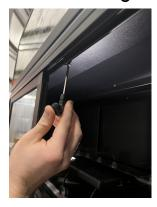
STEP 6: Attach the included male to male barrel connector into the top of cabinet and back of sign as shown.
